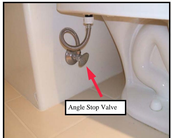
These valves need to be exercised. The plastic pipe is behind the valve inside the wall. If the valve handle does not turn easily, the plastic can break.
